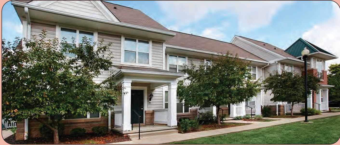
BELOW: New Pennley Place buildings are slated for extensive renovations in East Liberty. The Community Builders, a local non-profit, plans to upgrade the kitchens, HVAC units, and elevators this year. Photo courtesy of Elizabeth Sensky.
