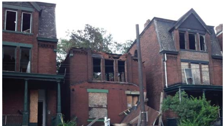
ABOVE: Three of the houses in historic Bride’s Row were severely damaged by fire on July 21. The owner of 5443 Penn Ave. (center) is Henry Enyenihi; 5441 and 5445 Penn are owned by Friendship Development Associates. At press time, the cause of the fire was unknown. Photo by Rick Flanagan
