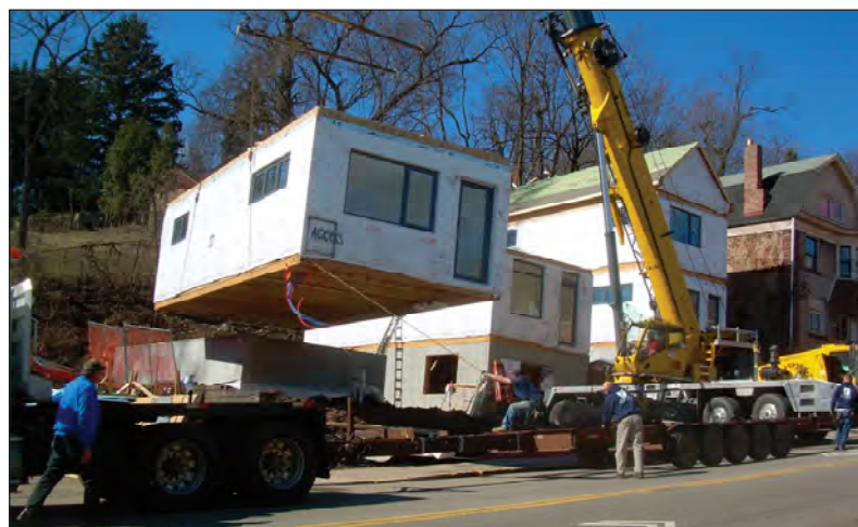
ABOVE: Workers lift a module into place, stacking progress on the construction of a house at 5456 Black St. Two single-family homes and a duplex are now being offered for sale by Module Housing, LLC. Photo by Rick Swartz.
